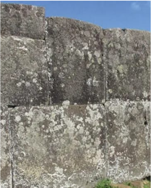
AHU NAU NAU AT ANAKENA BEACH · VINAPU MEGALITHIC WALL — AARON HYNES
